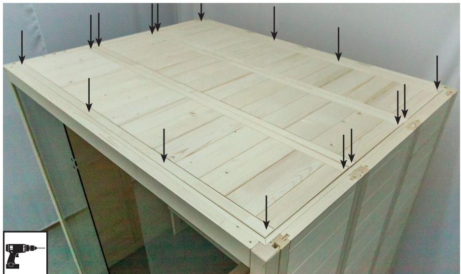
3 mm drill bit, 16 screws 4 x 70 mm
