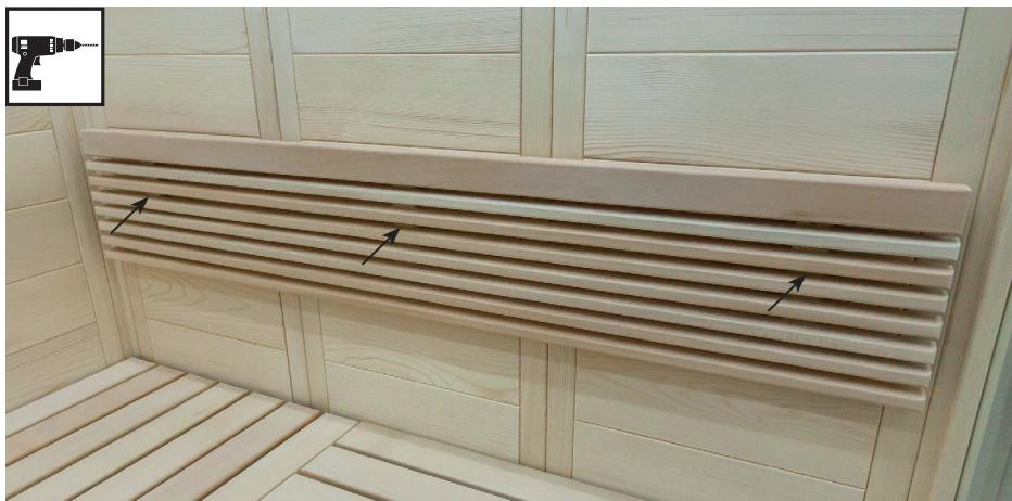
3 mm drill bit, 3 screws 3 x 40 mm
