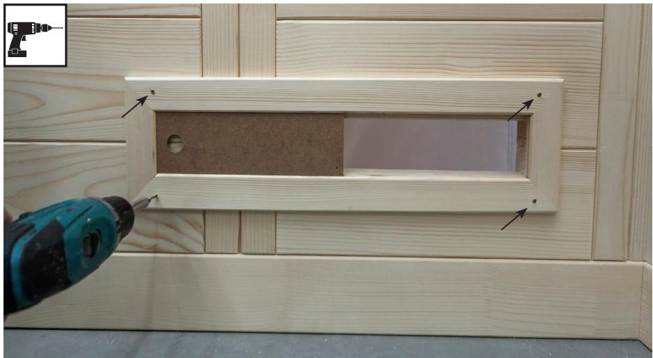
3 mm drill bit, 4 screws 3.5 x 40 mm
