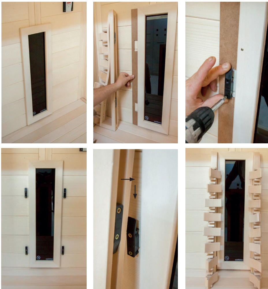
Fig. 29: Installing the backrests
