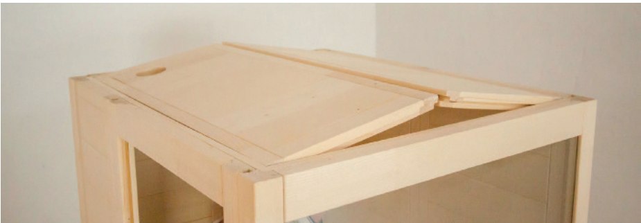
Fig. 15: Fastening the ceiling elements
