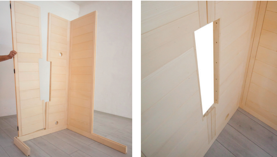
Fig. 6: Inserting wall element with recess
