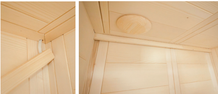
Fig. 24: Attaching the LED strip
