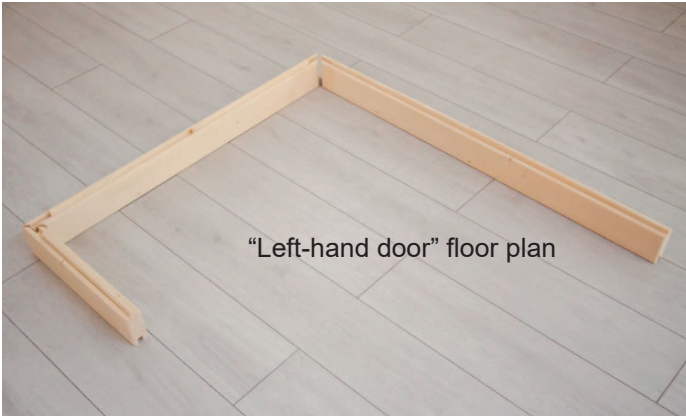
Fig. 1: Laying the three base frame elements
