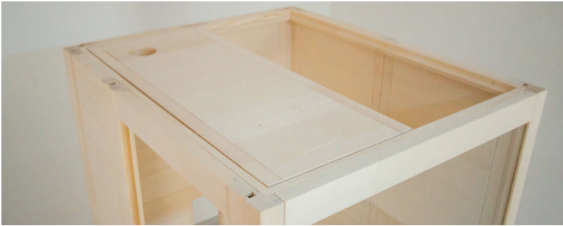
Fig. 14: Inserting front ceiling element
