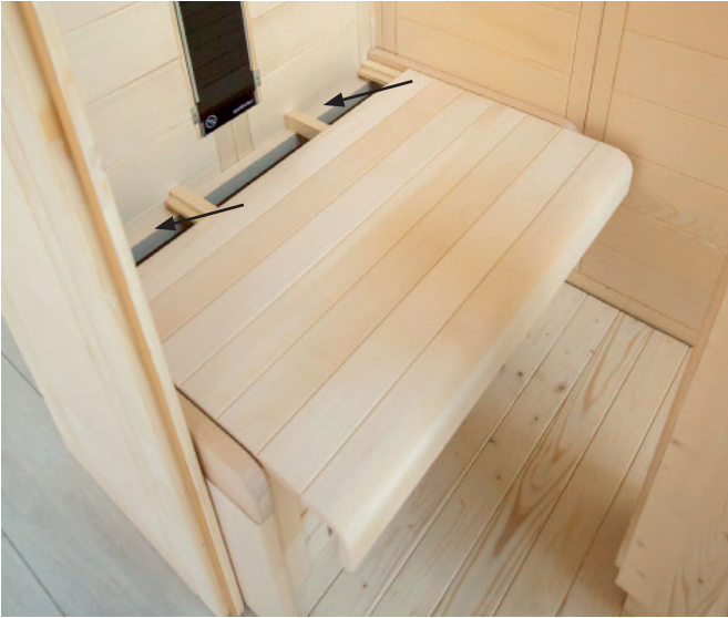
Fig. 28: Attaching the bench
